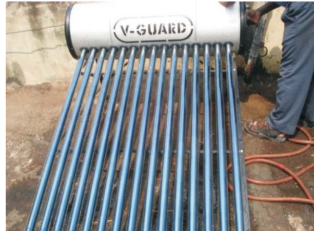
Fig. 4. Solar collector and solar tank
